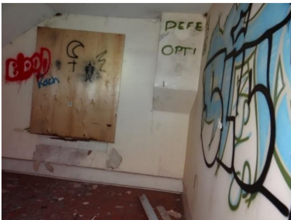
Plate 40: Bedroom in the addition on the second floor.
