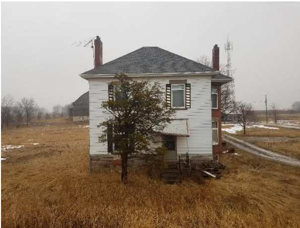
Plate 12: House, featuring vinyl siding, facing east.
