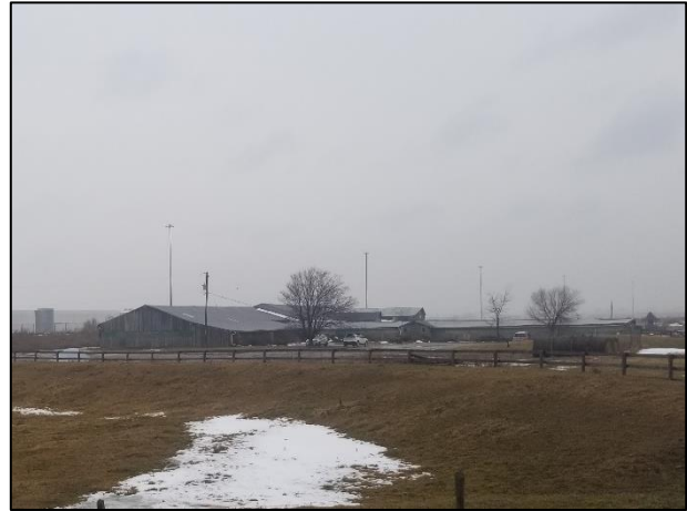
Plate 6: Complex of stables looking northeast towards the “original” portion (left) and addition extending south (right).
