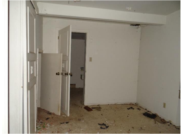
Plate 23: Main floor bedroom, looking north west
