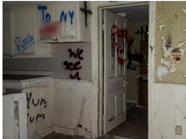
Plate 27: View to the western room adjacent to the kitchen*.
