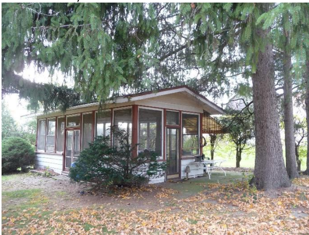
Plate 22: Summer house looking northwest (Town of Oakville 2014).
