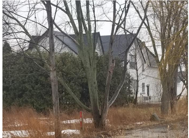
Plate 13: View of the north elevation, looking southwest from the driveway
