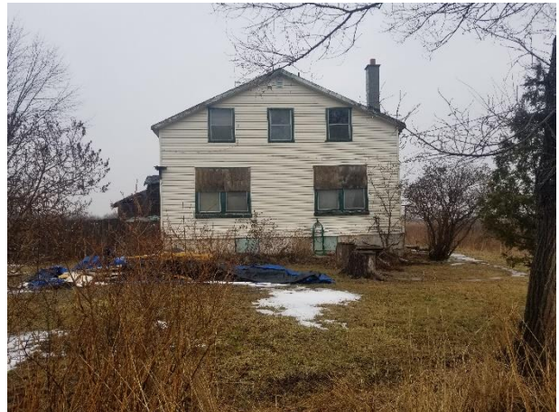
Plate 8: West elevation of the residence facing east.
