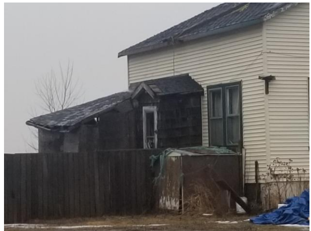
Plate 12: Frame additions on north elevation with north entrance, looking east. Note the fencing enclosing the storage area to the north and east of the residence.
