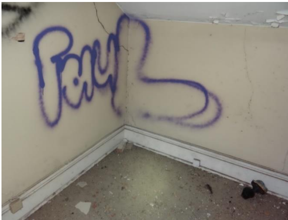
Plate 42: Detail of carpeted flooring and the tall baseboards.
