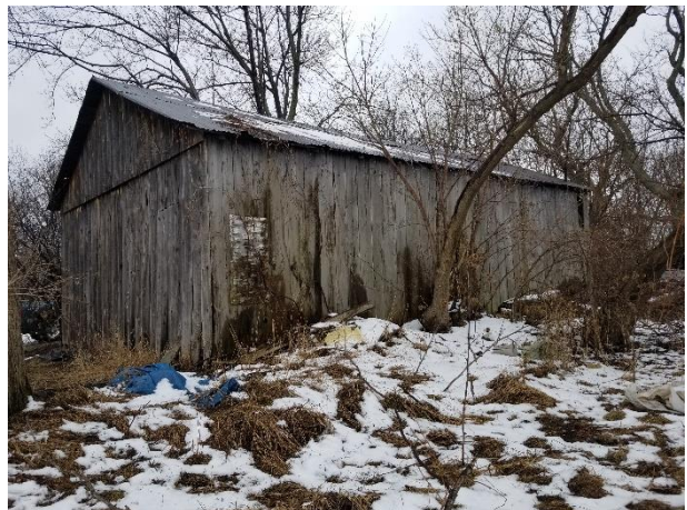
Plate 12: South and east elevations of the east outbuilding
