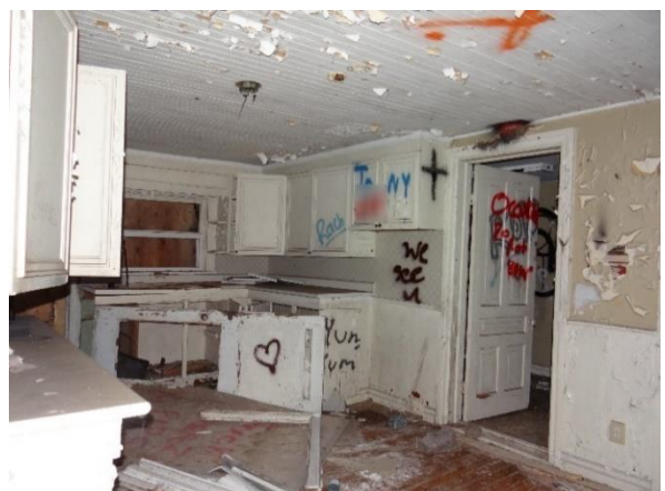
Plate 25: Kitchen in the northern addition*.
