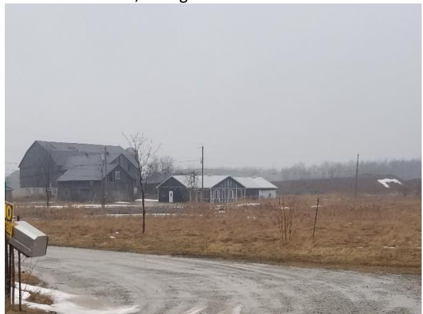
Plate 23: Barn, driveshed, and sales shop/storage facility, facing northeast.
