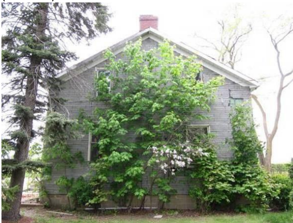
Plate 16: West elevation of the farmhouse, looking east (ASI 2010).
