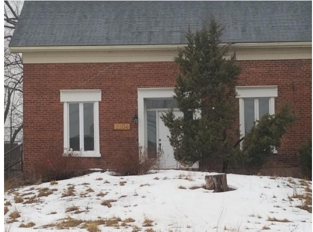
Plate 9: Detail of the front elevation, the replaced windows, and the vinyl fascia under the eaves (March 2020).
