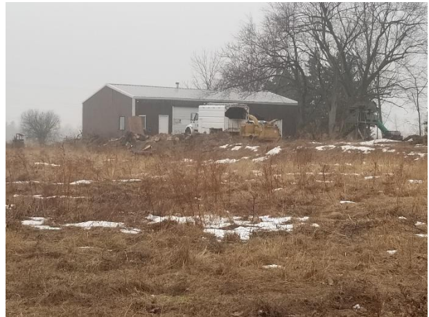
Plate 11: View of the garage, southwest of the house (March 2020).
