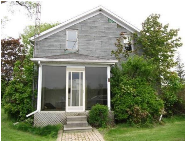
Plate 14: East elevation of the farmhouse, looking west (ASI 2010).
