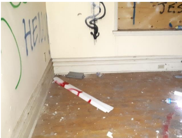
Plate 22: Detail of tall baseboard and wood flooring.
