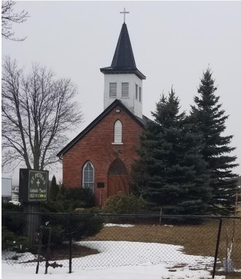
Plate 6: Front (east) elevation.
