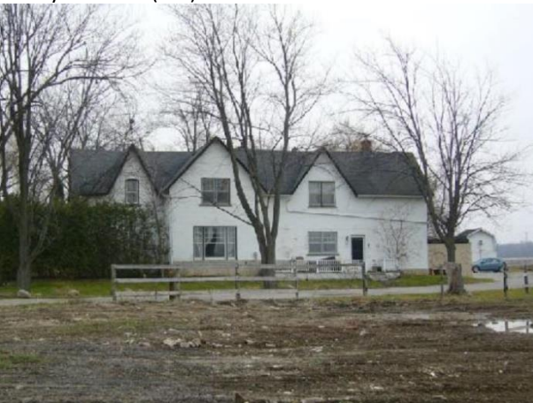
Plate 16: North elevation of the residence (Cuming 2016).
