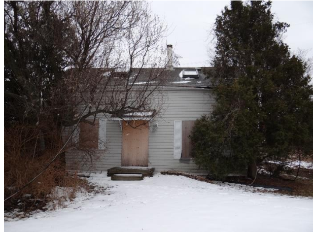
Plate 9: North elevation (log house portion)
