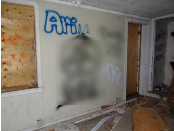
Plate 16: Large room in the original portion of the house*.
