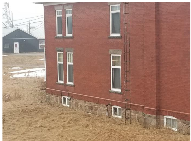
Plate 19: Symmetrical windows with lintels and sills, north elevation.
