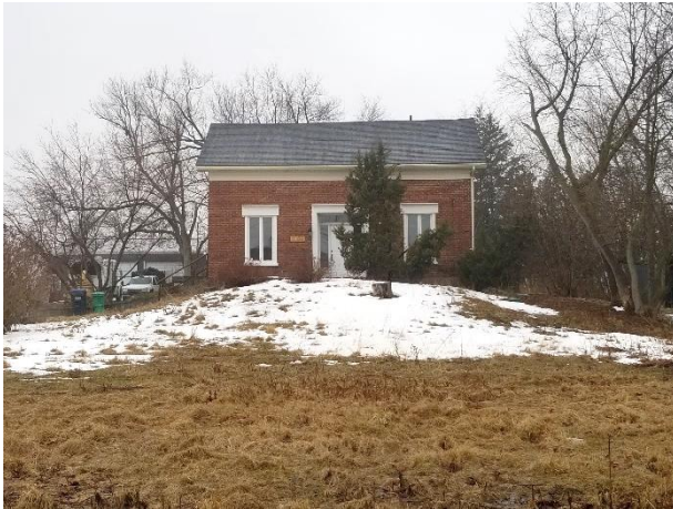
Plate 6: View of the northeastern elevation (March 2020).
