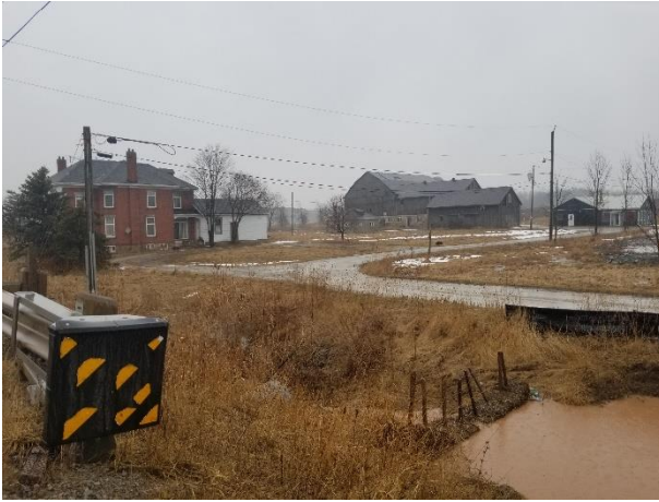
Plate 10: House and barns, facing northeast.
