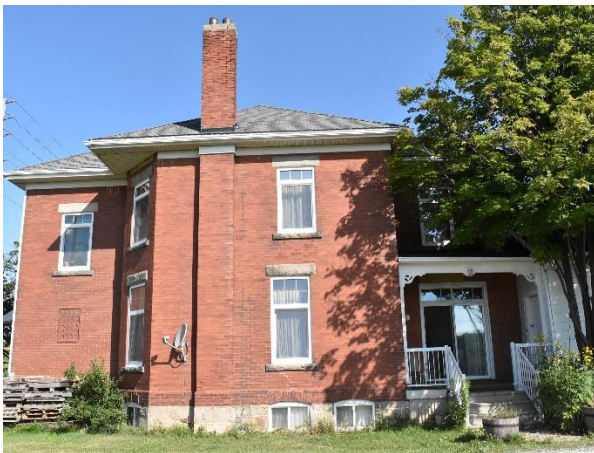
Plate 16: Main entrance, up stairs next to tree (Town of Oakville, 2018).
