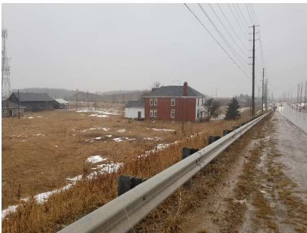
Plate 8: Embankment supporting Sixth Line, facing south.
