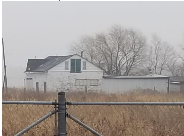
Plate 15: View south of the garage and rear addition.
