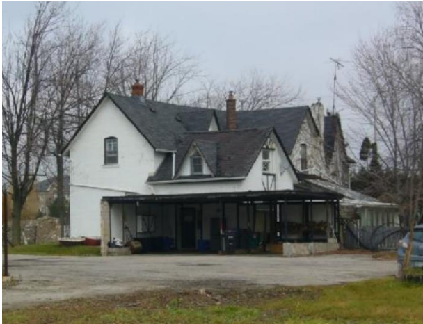
Plate 24: West elevation with gable end of nineteenth-century structure at left and later addition to the right (Cuming 2016).
