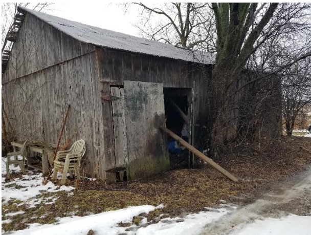
Plate 11: North and west elevations of the east outbuilding
