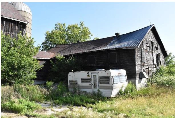
Plate 24: Barn extension and silo, facing northeast (Town of Oakville, 2018).
