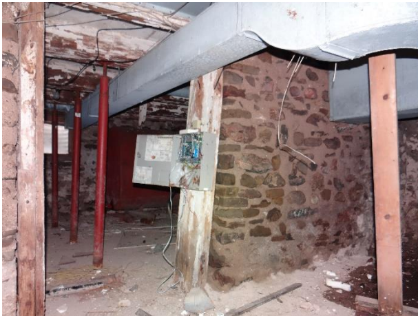
Plate 18: View of the basement looking west.
