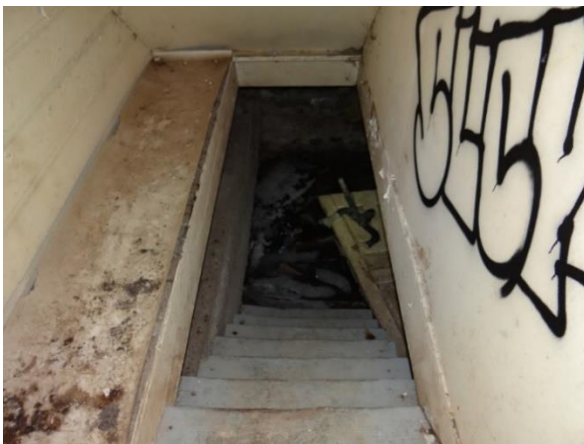
Plate 28: View from the main floor down to the basement.
