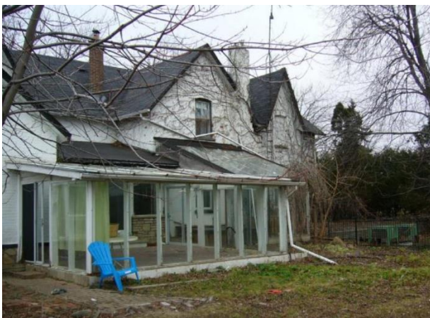
Plate 22: South elevation of the residence featuring sun room addition (Cumings 2016).
