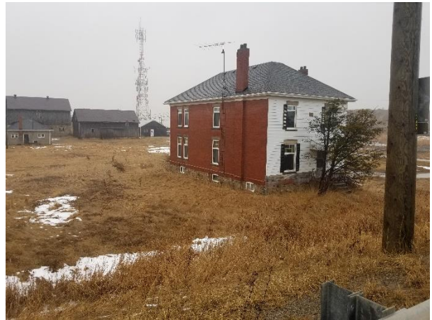
Plate 13: House, with barns, outbuildings, and cell tower in behind, facing southeast.
