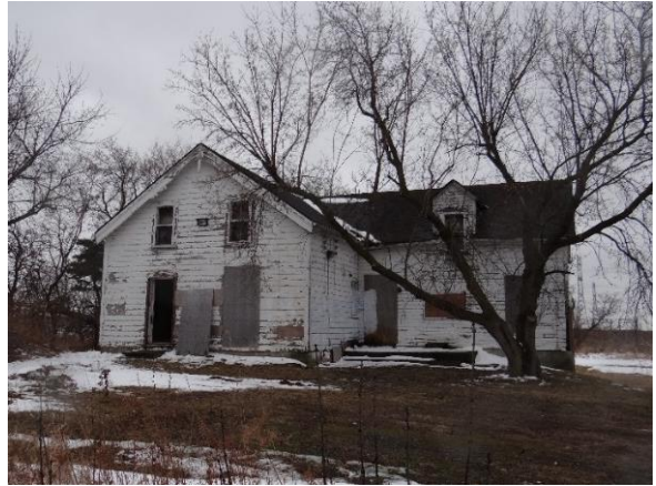
Plate 9: Farmhouse, east elevation.
