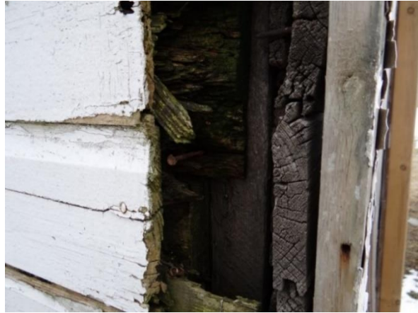
Plate 11: Wooden siding over original structure.
