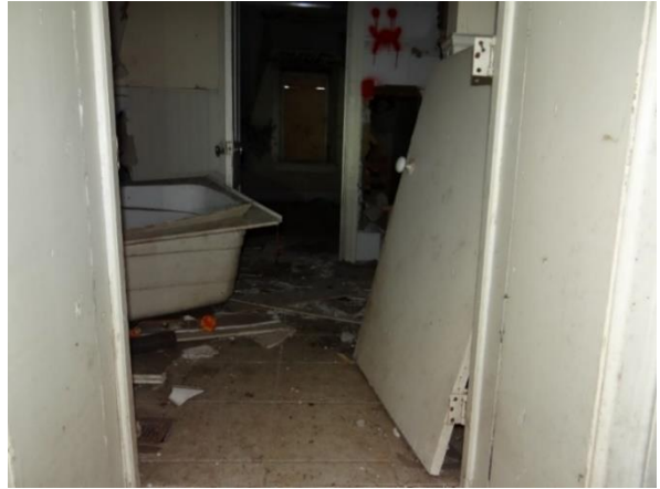
Plate 33: View into the bathroom in the original structure.
