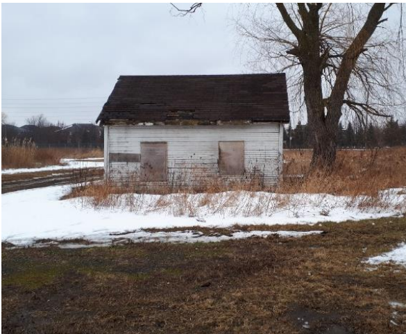
Plate 12: Garage, west elevation.
