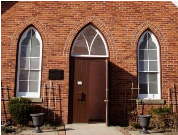
Plate 8: Detail of the entryway and windows on east elevation. Date unknown (Anonymous 2019).
