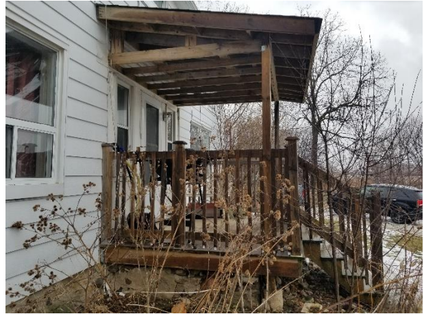
Plate 6: Covered front porch, parged stone foundations are visible in the photo
