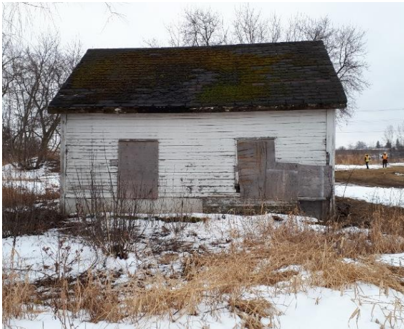
Plate 14: Garage, east elevation.
