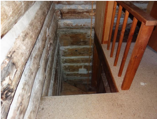
Plate 14: View looking down stairwell, looking south, note the rounded logs
