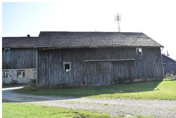
Plate 25: Driveshed, facing east (Town of Oakville, 2018).
