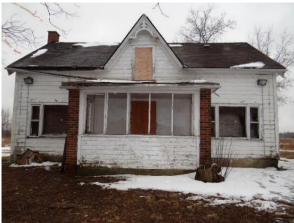
Plate 6: Farmhouse, south elevation.
