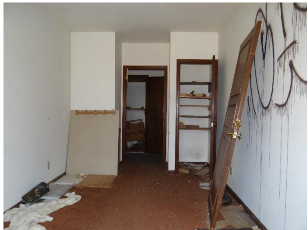
Plate 25: Former kitchen, looking north
