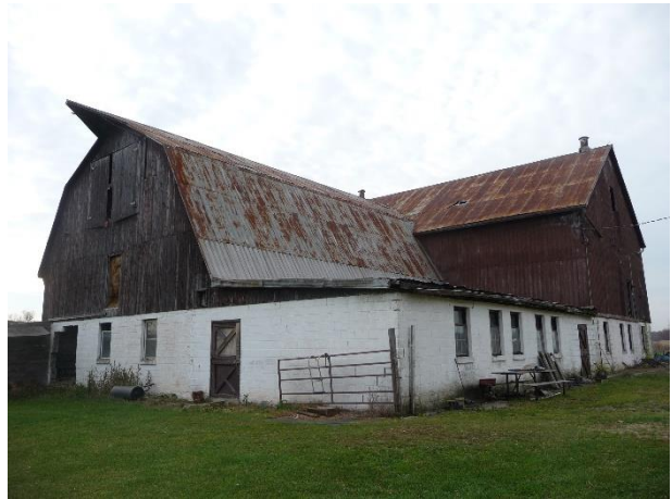
Plate 19: Barn complex showing gambrel addition (left), one-storey flat roof addition (centre) and heavy timber bank barn (right/rear) (Town of Oakville 2014).
