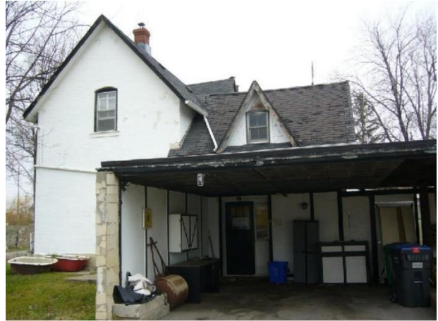
Plate 25: West elevation with addition and lean-to car port. West elevation of original residence at left (Cuming 2016).
