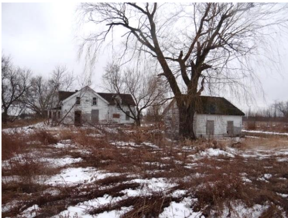
Plate 2: View of the property and garage, looking west.
