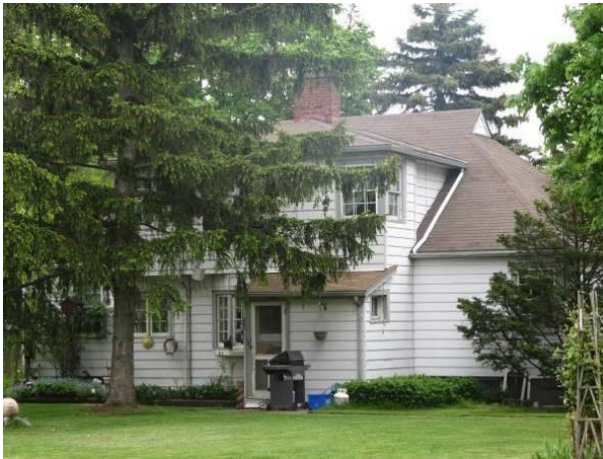
Plate 18: North elevation of the twentieth-century dwelling, looking southwest (ASI 2010).
