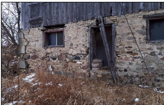
Plate 24: Detail of the barn's stone foundation
