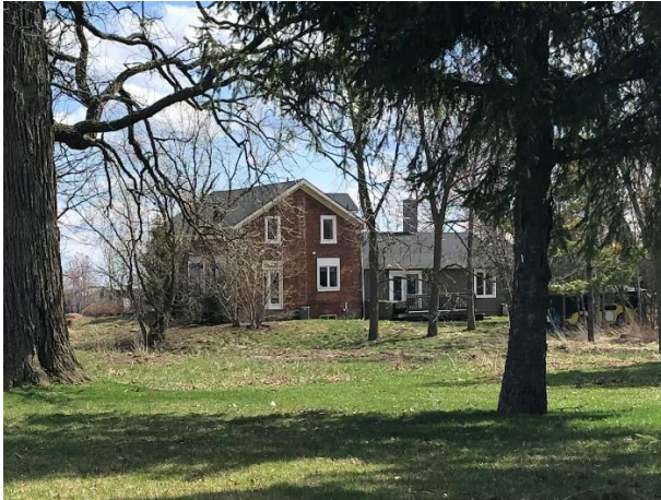
Plate 8: View of the northwest elevation (April 2020).
