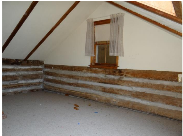
Plate 17: View of large west bedroom, log house second floor
