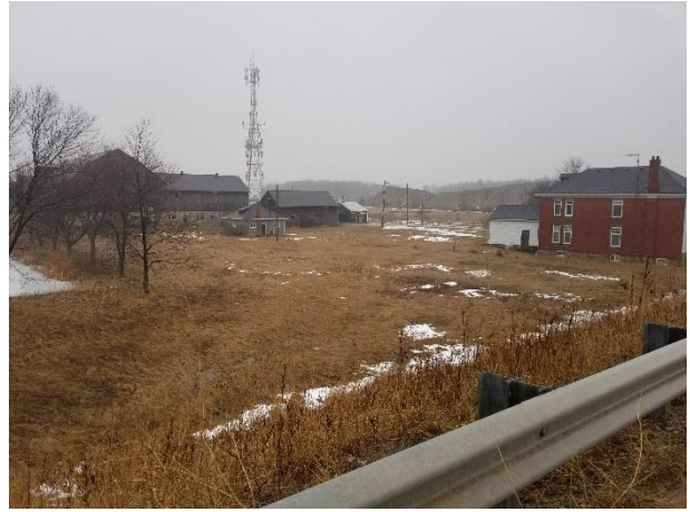
Plate 11: House, barns, outbuildings, and cell tower, facing southeast.
