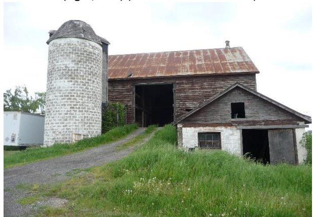
Plate 21: North elevation of barn complex showing silo (left) bank barn (centre) and smaller gable roof shed addition (right)(Town of Oakville 2014).
