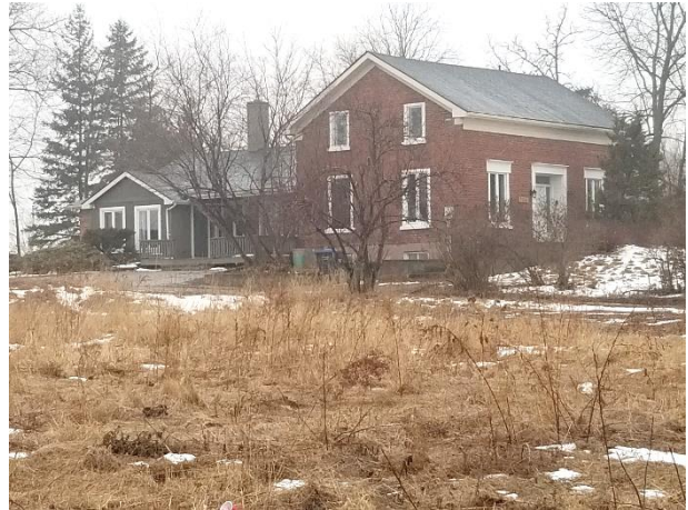
Plate 7: View of the southeastern elevation and rear addition (March 2020).
