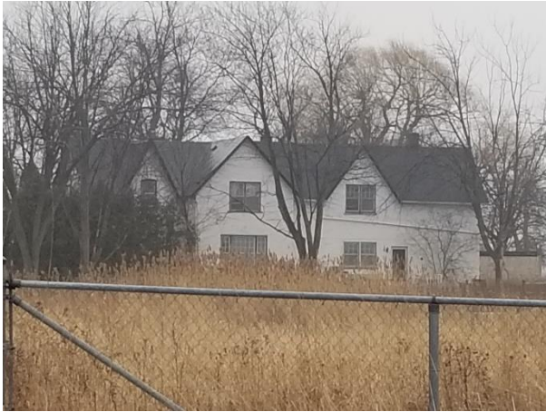
Plate 12: North elevation of the residence, looking south.
