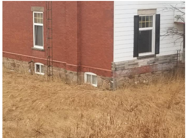
Plate 15: Stone foundation, north elevation.
