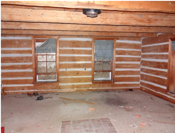
Plate 10: View of log house main floor, looking west
