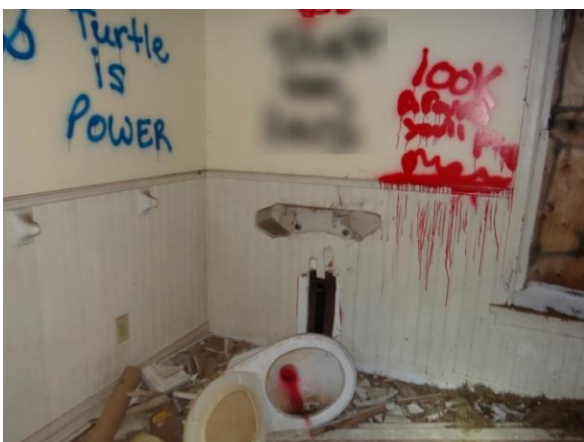
Plate 24: Toilet in the bathroom, note the wood panels along the wall*.
