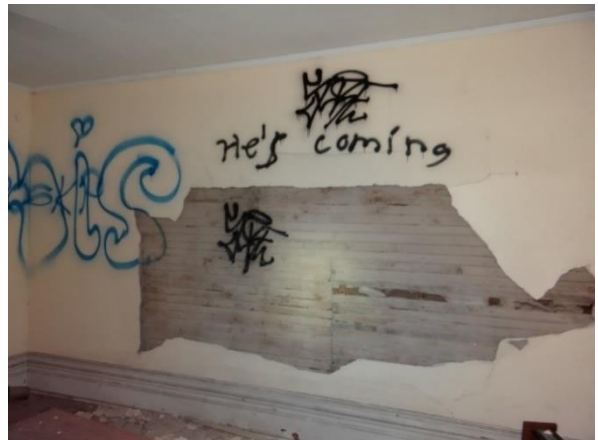
Plate 19: Bedroom on the main floor.
