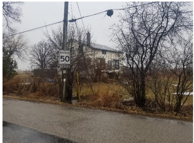
Plate 10: South elevation and south yard, looking northeast.
