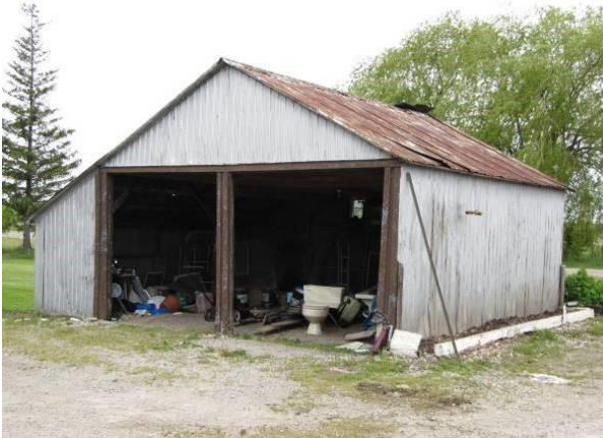
Plate 24: Frame shed/garage looking northwest from the driveway (ASI 2010).
