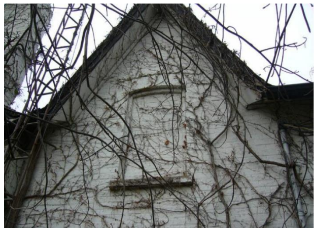
Plate 23: Bricked-in window on second floor of the south elevation (Cumings 2016).
